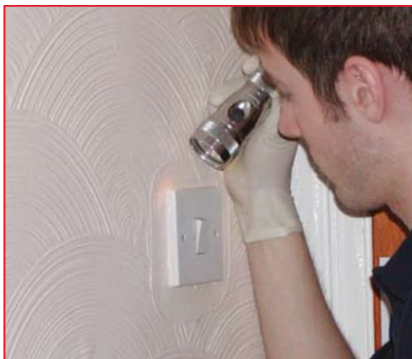
• Remove and inspect light switch covers
